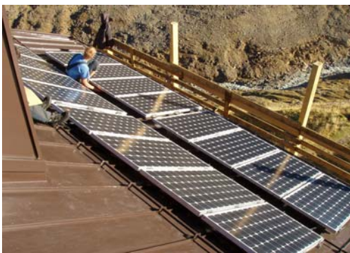
Photovoltaikanlage 3 kW
